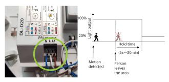
For 20% standby ensure blue wire is in "N" terminal, white wire in "L" terminal and brown wire in "L1" terminal.
