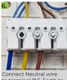
Connect Neutral wire to terminal "N", Earth to Earth terminal, Active wire to terminal "1"
