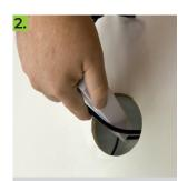
Pass the driver and battery pack through the cutout and secure it in place. Guide the cable through the cutout and connect to mains power. Ensure the battery is connected.
