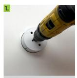
Mark the position on the ceiling and create a 75mm-150mm diameter cutout.
