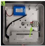
Run cables into the fitting and connect to terminal block
